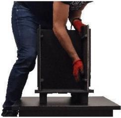
2. Place the stove base (1) on a flat surface. Apply a 3-4 mm thick layer of heat-resistant sealant on the base at the wall fixing points. Apply sealant to the vertical grooves in the back wall (3). Install first the side wall (2), then the back wall (3) and finally the remaining side wall (4) firmly to the base.
