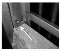
Once the front soapstones have been installed, place the stones meant to be inside the heater (approx. 30kg). Some stones also have to be placed on the heating elements.
