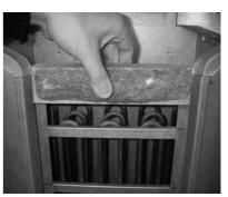
Install the intermediate pieces (8) of the soapstones so that the projection will always stay on the stone i.e. there will always be an air gap between the stones.
