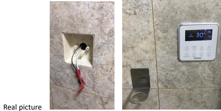
Figure 9 Controller installations
