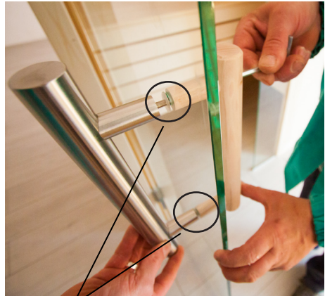
Attach plastic washers on the stainless steel handle
